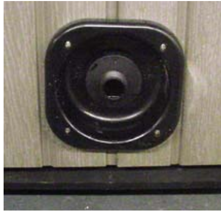
Figure 13. Cabinet mounted drain valve
